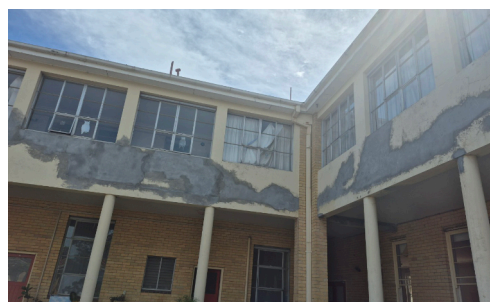
Above and left: the walls and concrete pillars facing the courtyard were pitted with 'concrete cancer', since cleaned and rendered thanks to donations from the School Building Fund. Below: the new pergola in the courtyard enables teachers and students to enjoy sitting outdoors.
