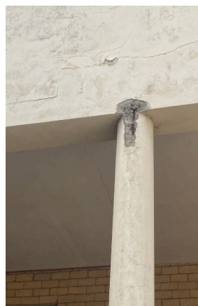
Above and left: the walls and concrete pillars facing the courtyard were pitted with 'concrete cancer', since cleaned and rendered thanks to donations from the School Building Fund. Below: the new pergola in the courtyard enables teachers and students to enjoy sitting outdoors.
